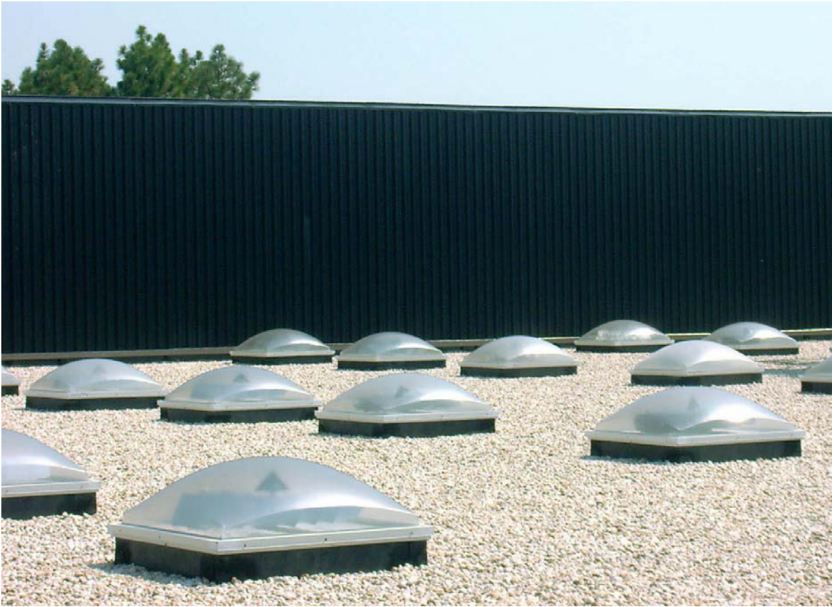
Figure 3.1.1 (left) Transpired collector mounted on south side of fabric warehouse
