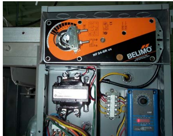
Figure 3.1.2 (left) Air distribution fan and flexible fabric duct which delivers air at ceiling. Figure 3.1.3 (right) Original fan controls which regulate outlet temperature with modulating damper.
