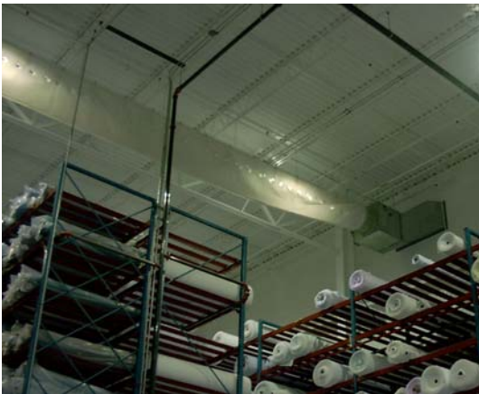
Figure 3.1.2 (left) Air distribution fan and flexible fabric duct which delivers air at ceiling. Figure 3.1.3 (right) Original fan controls which regulate outlet temperature with modulating damper.
