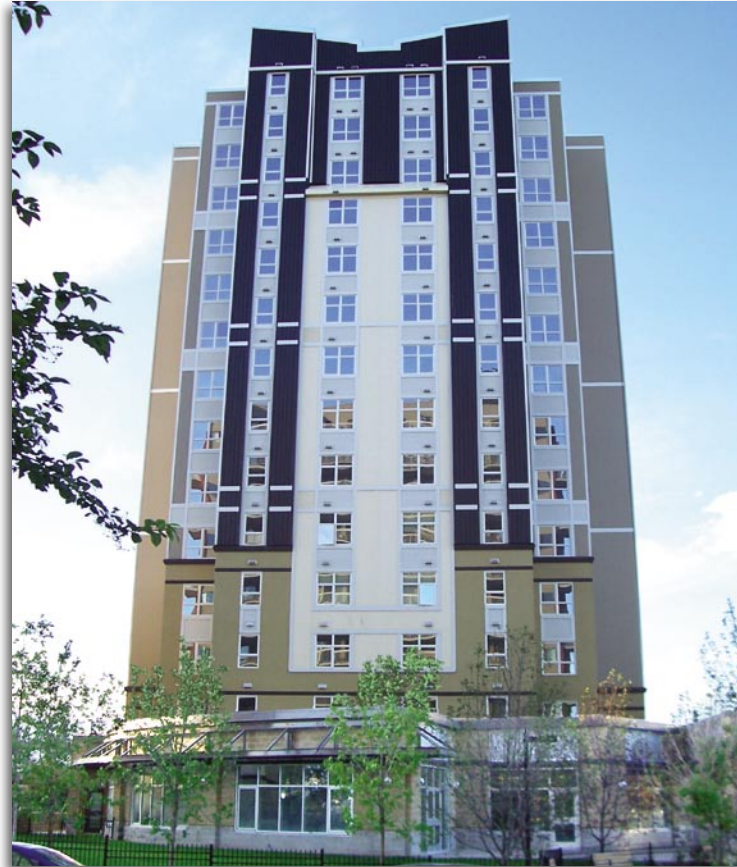
▲ Long, narrow SolarWall panels are a dramatic feature of this Calgary, Alberta apartment complex.
