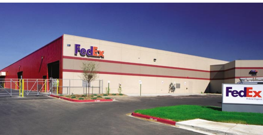
◀ Federal Express distribution center, Colorado: Dark red SolarWall panels span entire southern wall.
