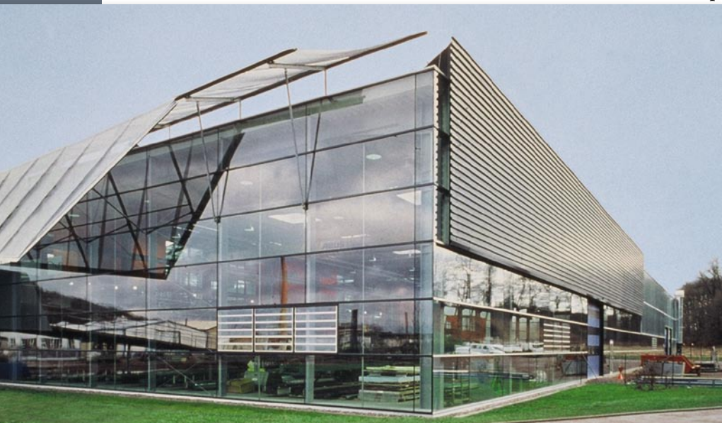
◀ Horizontal SolarWall panels, German manufacturing facility.
