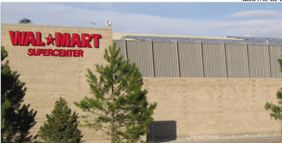
◀ SolarWall panels on a Wal-Mart in Colorado.
