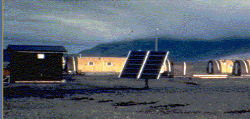
Parks Canada PV-Wind Hybrid System (Arctic at 81°N)
