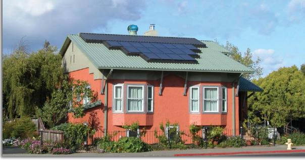
Of greater concern is that the heat build-up can damage PV cells, shortening their useful life. In some cases, roof temperatures get so hot that the underlying roofing materials get damaged, too. How hot? Temperatures of over 85°C have been recorded on bright summer days – not exactly great news for shingles or building managers.
