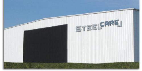
Through the relatively simple step of converting the 30,000 square feet (2,787 m²) hangar doors to a solar heater, and using SolarWall technology on an existing south wall to preheat outside air and improve air flow, the problems were solved. Ceiling and exhaust temperatures fell to within 3° F (1.5° C) of the floor temperatures, evening out both heating and humor. No more negative air pressure equals no more drafts which equals no more negative employee and union pressure.
