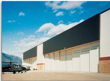
much as they were looking to save on energy costs. The same holds true in Fort Carson where the SolarWall system helps to combat the fume-related challenges inherent with maintaining diesel-fueled helicopters and other military vehicles. In both cases, thanks to their SolarWall installations, these base buildings now have plenty of fresh air.
