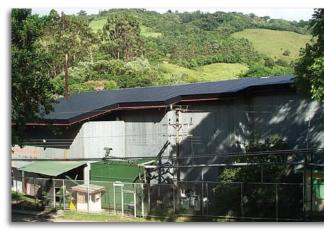
A "nitty-gritty" finale: SolarWall panels work well with tunnel, trough, conveyor and other types of driers; existing operations can be easily converted to include solar heating of the air being directed to the drier intake fans. The all-metal panels are installed on either the roof or a nearby wall and the system is then connected to the drier fan intake. All the air passes through the solar panels first, where it is pre-heated before being directed to the drying chamber.
