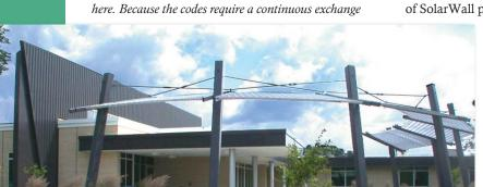
of a significant portion of the building's air, you have to run the heating system overtime to recover the heat. For all the cold air you bring in, you've thrown away just as much hot air. By using SolarWall to pre-heat the incoming air, you get rid of the whole BTU trading process – it just goes away. That's a huge savings; it's like free gas for your car.
