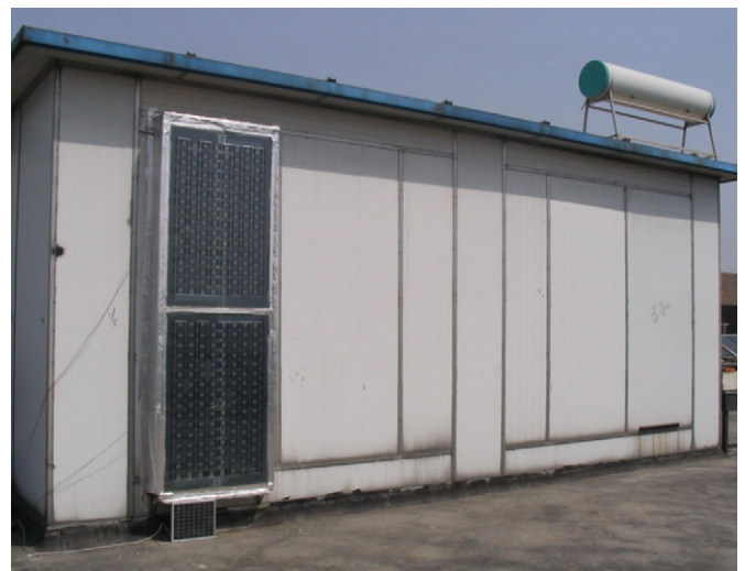
Fig. 2. Graphic representation of the PV-Trombe wall assisted with DC fan and hot-box.
