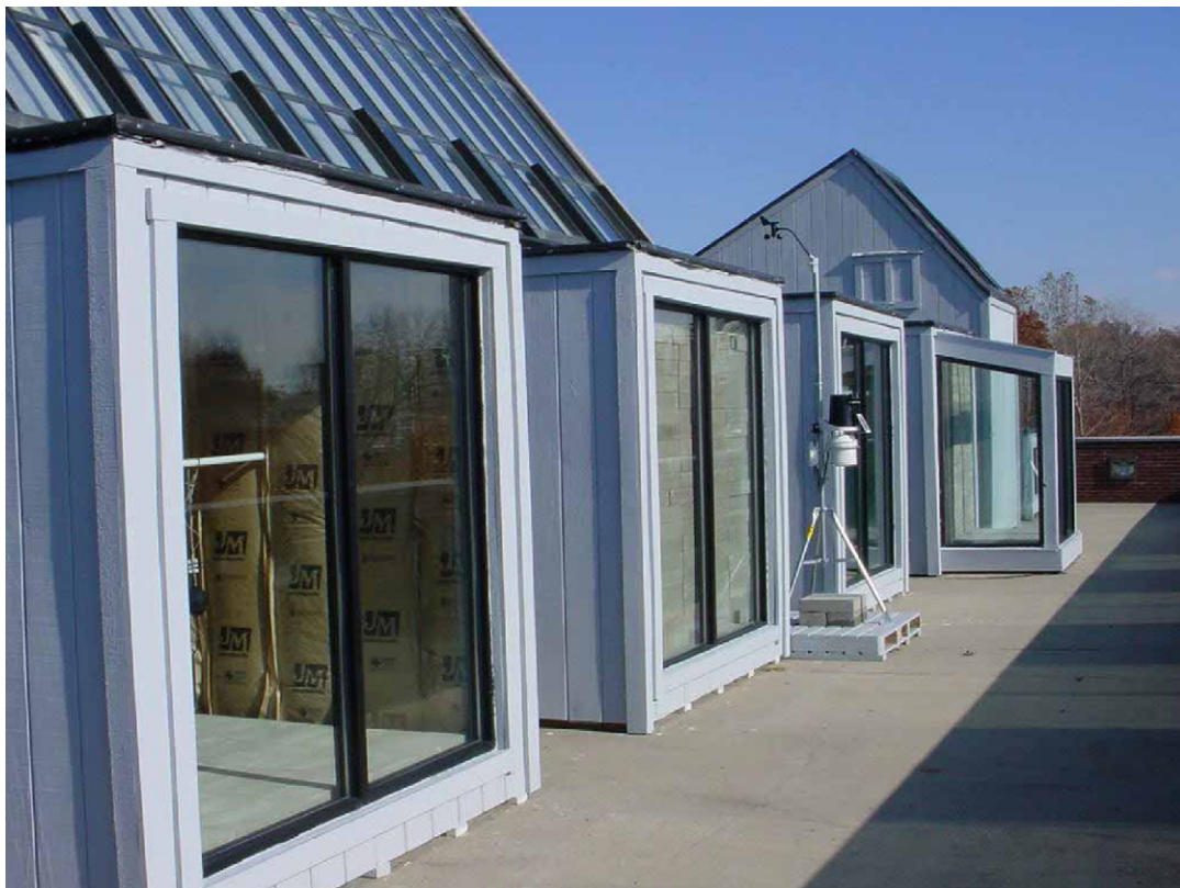
Fig. 1. South view of the five passive solar test-cells (from the left): Direct Gain (DG), Trombe-wall (TW), Water-wall (WW), Sunspace (SS), and Roofpond (RP).
