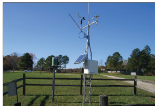
This station for the National Estuarine Research Reserve (NERR) in Virginia transmits data via our GOES satellite transmitter.
