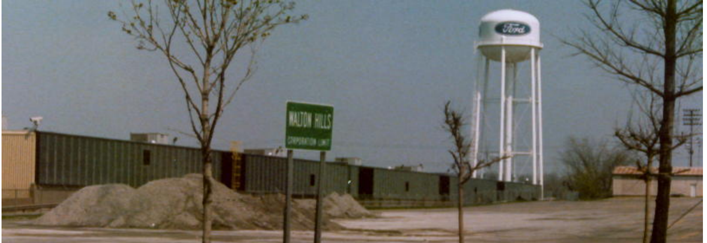
SolarWall® technology at Ford Walton Hills Stamping Plant near Cleveland, Ohio. This was one of seven North American stamping and assembling plants that installed SolarWall systems.
