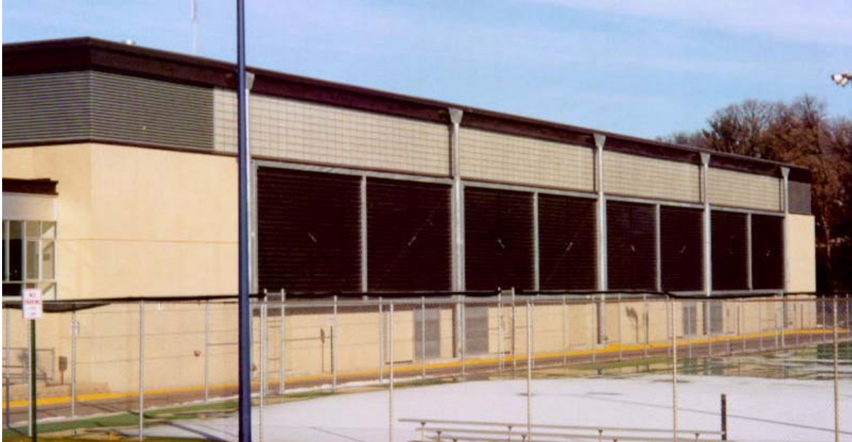
SOLARWALL® panels on south facade of private school
