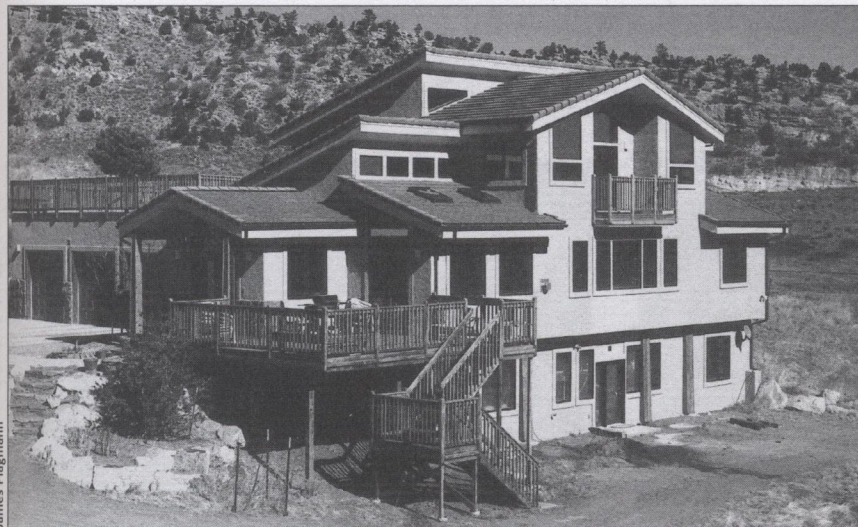
FIGURE 3-8 A direct-gain passive solar home. Sunlight streaming through south-facing windows is converted to heat inside the home, directly heating the interior space. This beautiful passive solar home in Morrison, Colorado, was designed by Colorado architect James Plagmann.
