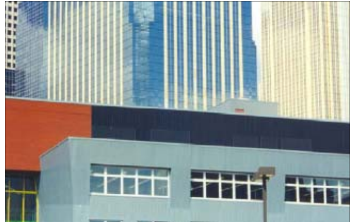
The black panels were integrated into a penthouse wall
