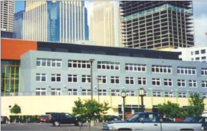
SolarWall® system at WMEP K-12 downtown school
