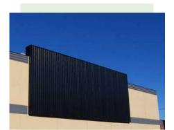
The passive solar wall draws warm air through it and into the building, cutting energy cost throughout the year.
